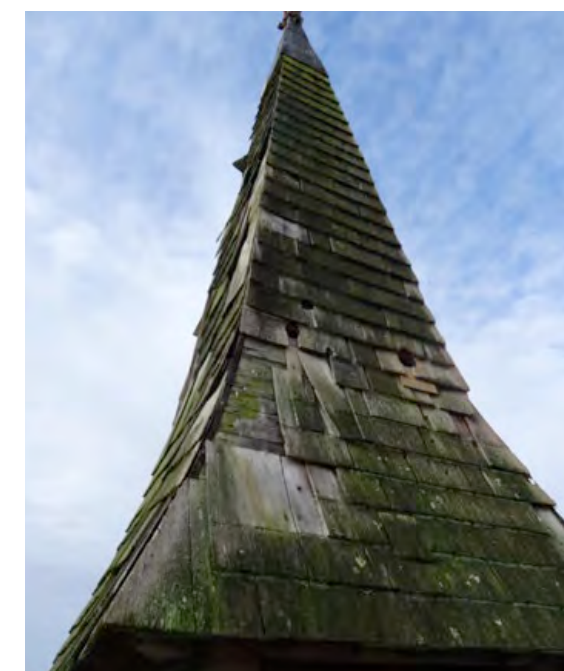
9. Cedar shingles indicative of re-shingling lost WWII. Woodpecker holes are indicative of inspect colonization of the spire.
