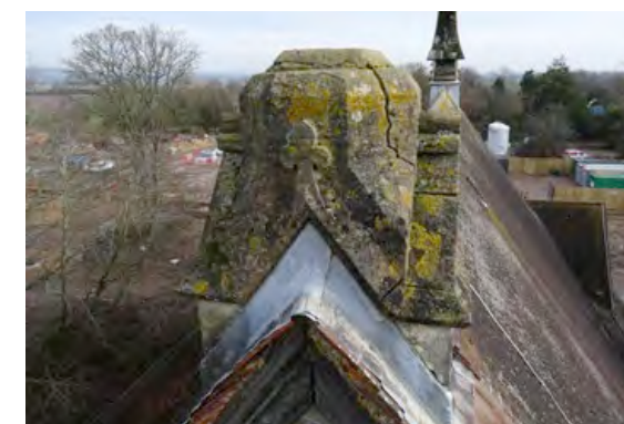
5. Portland stone chimney at head of West gable now devoid of pot.
